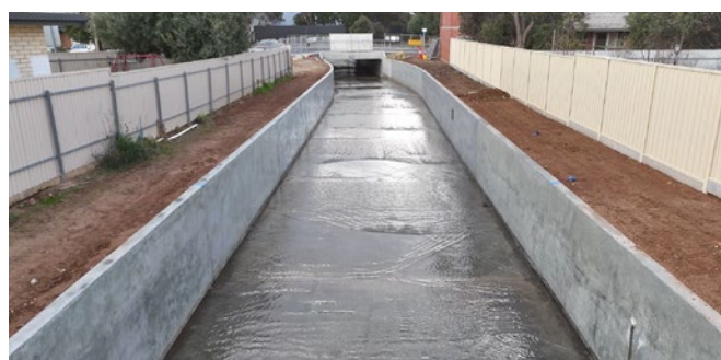
Channel construction through to completion
